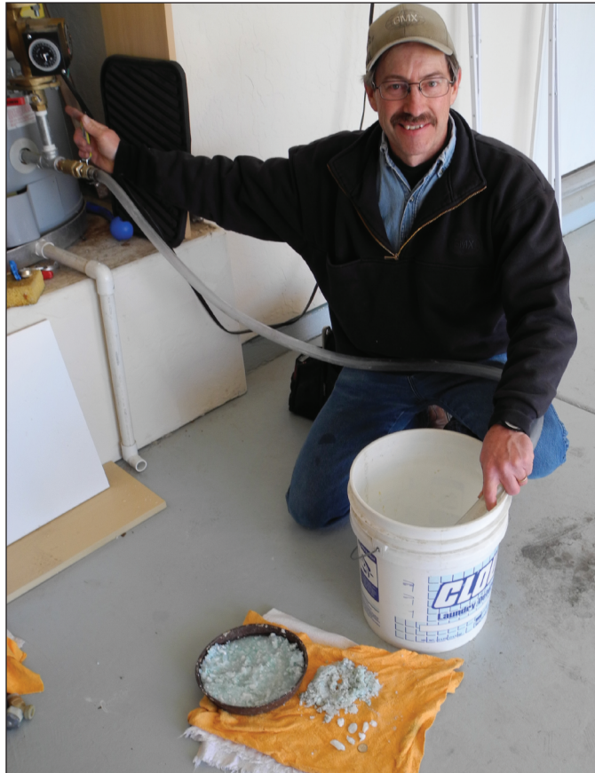
Hard water sediment builds up inside your hot water heater making it operate less efficiently. GMX magnetic technology treats hard water. Here, GMX distributor Larry Brown drains a water heater, collecting the bluish sediment (foreground).
