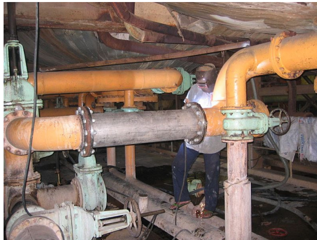
A new section of SS Pipe installed with flanges at the main inlet of Evaporator 4 for installation of 10 nos GMX 8000s
