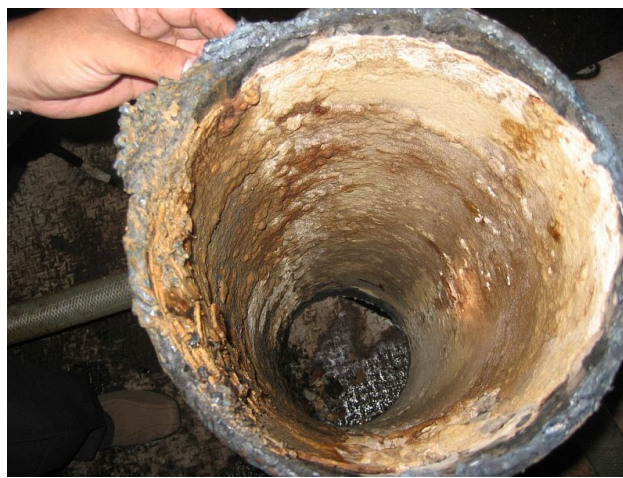
Inside view of the scaled main inlet to evaporator 4
