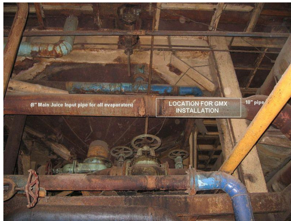
Location for GMX 8000 installation on main juice inlet for all evaporators
