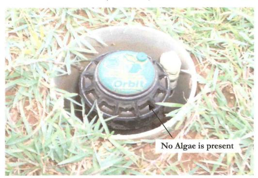
CONDITION OF STRAINER INSIDE THE SPRINKLER AFTER 10 DAYS OF INSTALLATION (WITHOUT GMX)
